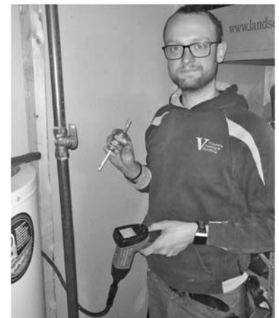
Here is Marvin performing a water heater inspection, shown here with his video inspection camera looking inside the water heater.
