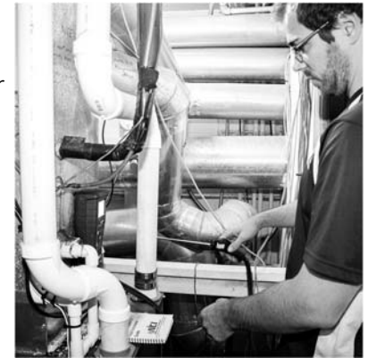
Brendan is checking his combustion analyzer on a furnace Combustion Optimization & Safety Inspection
